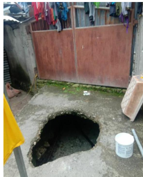
Current use of spring water outside the existing distribution network
